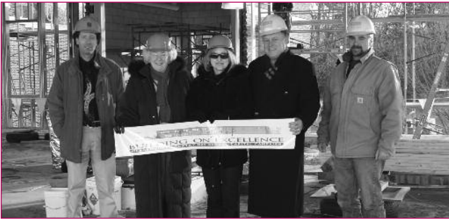
Architect Mark Humphreys; Principal Sister Martha Mulligan; Capital Campaign Co-Chairs Roseanne (Grinsell, '77) and Sam Simmons; and Construction Manager Peter Fiore atop the second floor addition in early December. Photo courtesy of Lisa Lydon
